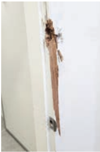
An inside door has been completely ripped from the lock inside the recently opened restaurant.
